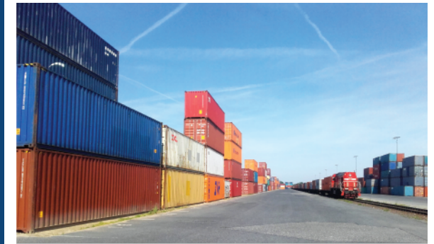
RAIL HUB TERMINAL GADKI (Poznan / PL)
